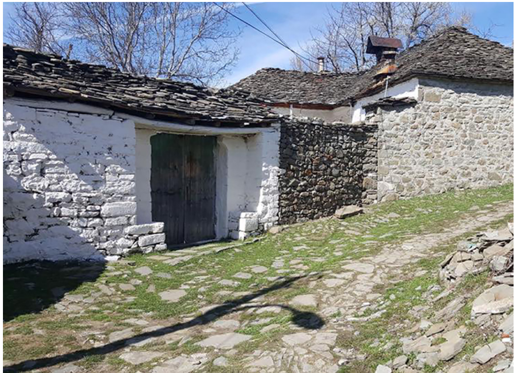
Fig. 6. Stone benches that allow the seat at the two side of the gate.
