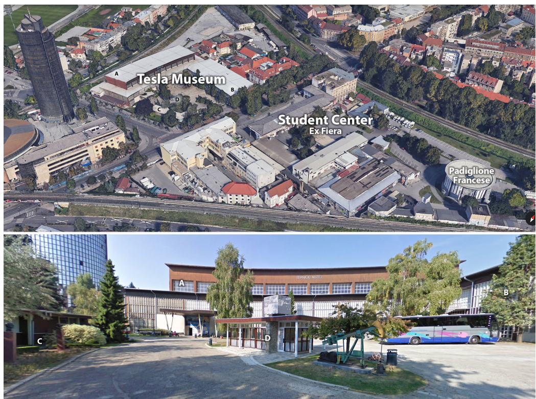
Fig. 1. Aerial view of the complex of the area of the former Zagreb Fairground realized on the basis of the project by Marijan Haberle and Hinko Bauer. The French pavilion, the student centre and the Tesla Museum are highlighted. The picture below shows the "square" at the entrance to the Museum with the four pavilions.
