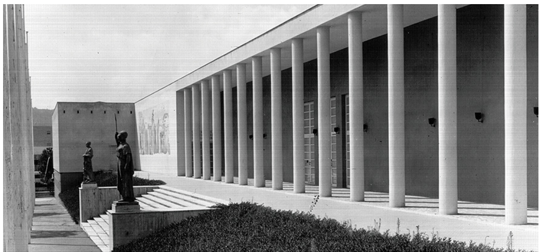
Fig. 3. Mostra d'Oltremare, Pavilion of Health, Race and Culture. Project realized by Ferdinando Chiaromonte, Naples, 1939-1940. Historical photo.
