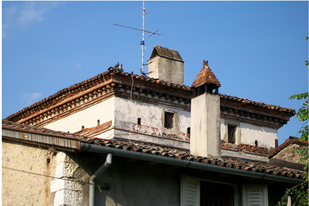
Fig. 4. Brick's practice in a dovecote tower located in Gussago (Bs).
