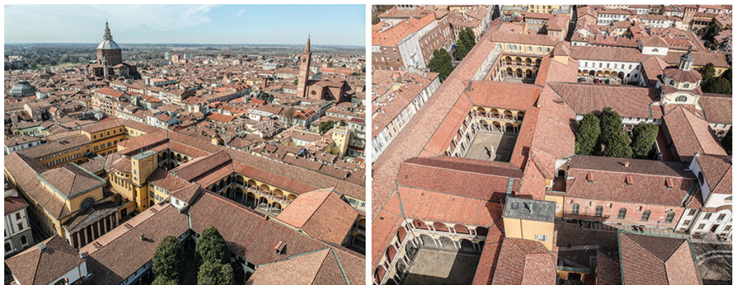
Fig. 1. Pictures of the Central Palace of the University of Pavia highlight its relationship with the layout of the historic core.
