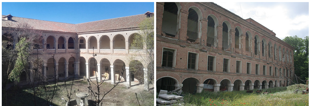
Fig. 3. Internal fronts turned towards the open spaces of the complex (court and rear garden).
