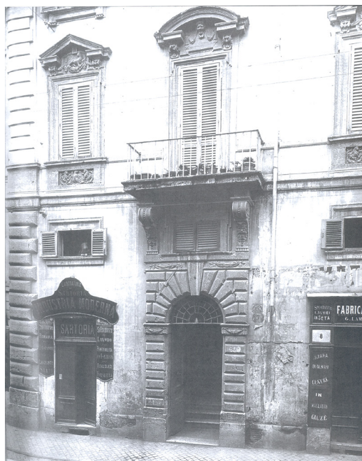
Fig. 2. Photograph of the building at n. 7 of Via Alessandrina before it was demolished [Delli 2007, vol. I].
