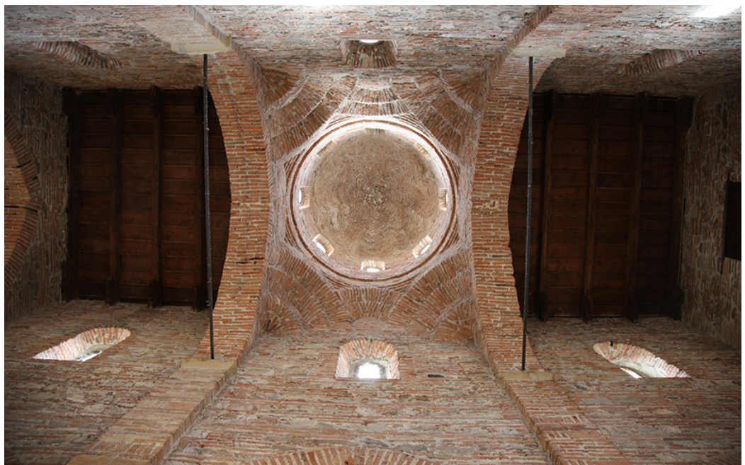
Fig. 2. The main dome of the central nave.
