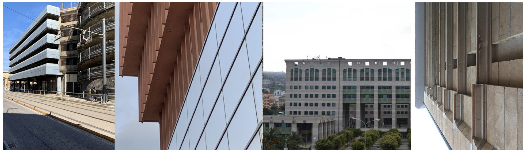
Fig. 7. Buildings and other equipment that reconfigure urban structures by strengthening the places of comparison between the cities on the Strait: the "Palacultura" or the palace of culture (Me), the Offices of the Region (RC), the Tram line (ME), the Airport (RC) (composition).
