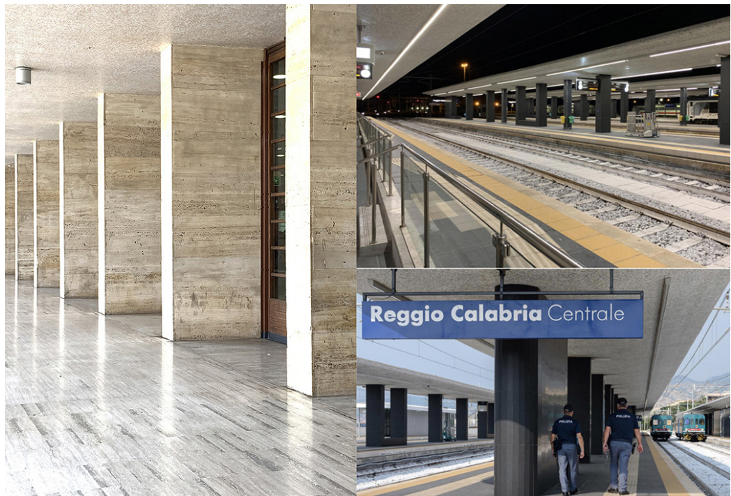
Fig. 1. The twin railway stations of Messina and Reggio Calabria, by Angiolo Mazzoni.
