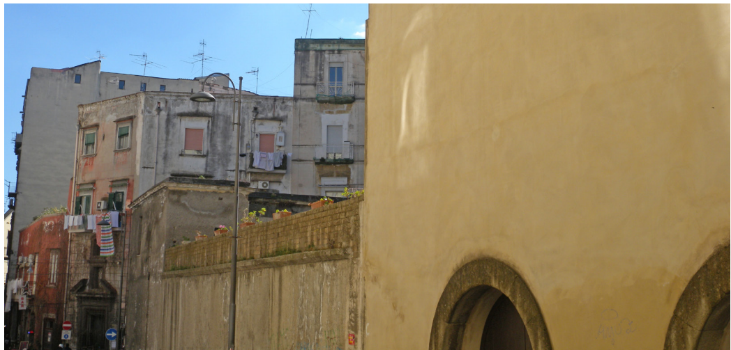
Fig. 7. The Monastery seen from Via Armani: the high irregular walls enclose the cloistered area, except for the space occupied by the former cloister, partially visible from the street.
