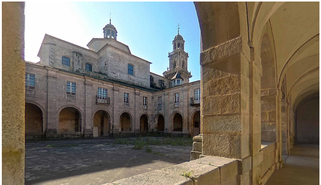
Fig. 12. Detail, from a 360° spherical panorama, of the cloister of the monastery of San Salvador de Lourenzá, Lugo, Spain (photo by the author 2019).
