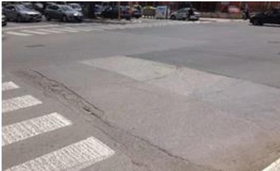
*Fig. 14.36: Pavement deformations at the North quadrant.*
