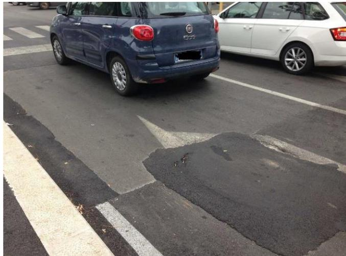
Fig. 14.31: Bad pavement condition on the turning lane in Viale Papa Giovanni XXIII, before the intersection with Viale O. Flacco.
