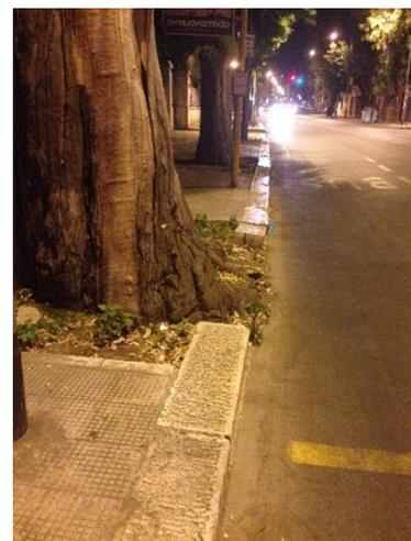
Fig. 14.32: Tree roots presence in the shoulders of Viale Orazio Flacco (near the intersection with Via Storelli).
