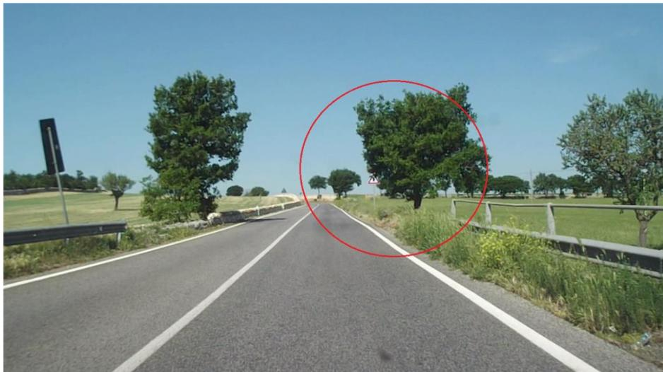
Fig. 13.11: Example of vertical traffic sign hidden by the trees.
