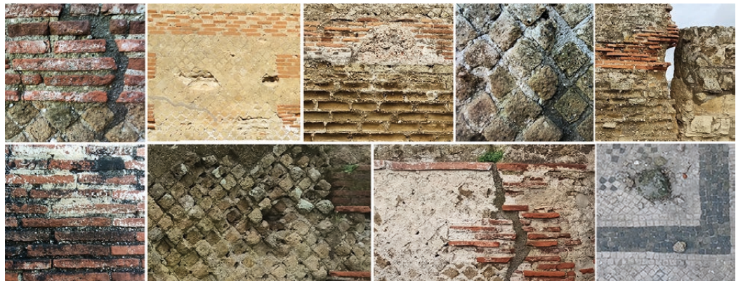
Fig. 2. Exemplificative framework of the variations and/or anomalies able to suggest the stratified structures in the various epochs.
