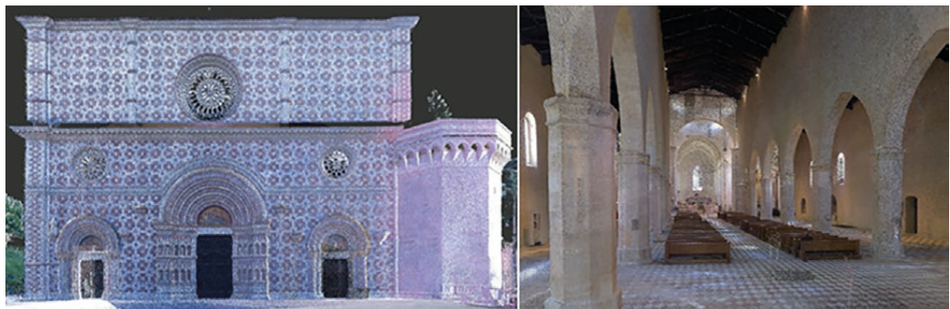
Fig. 1. Views of the point cloud of the Basilica of Collemaggio.
