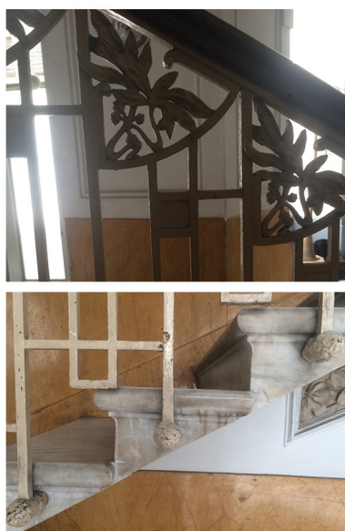
Fig. 5. Helicoidal staircase of Palazzo Mannajuolo. Detail of the design solution.
