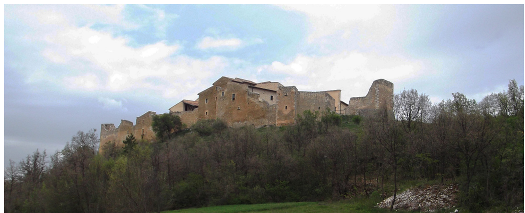
Panoramic view of Castel Camponeschi (AQ), (photo by authors).
