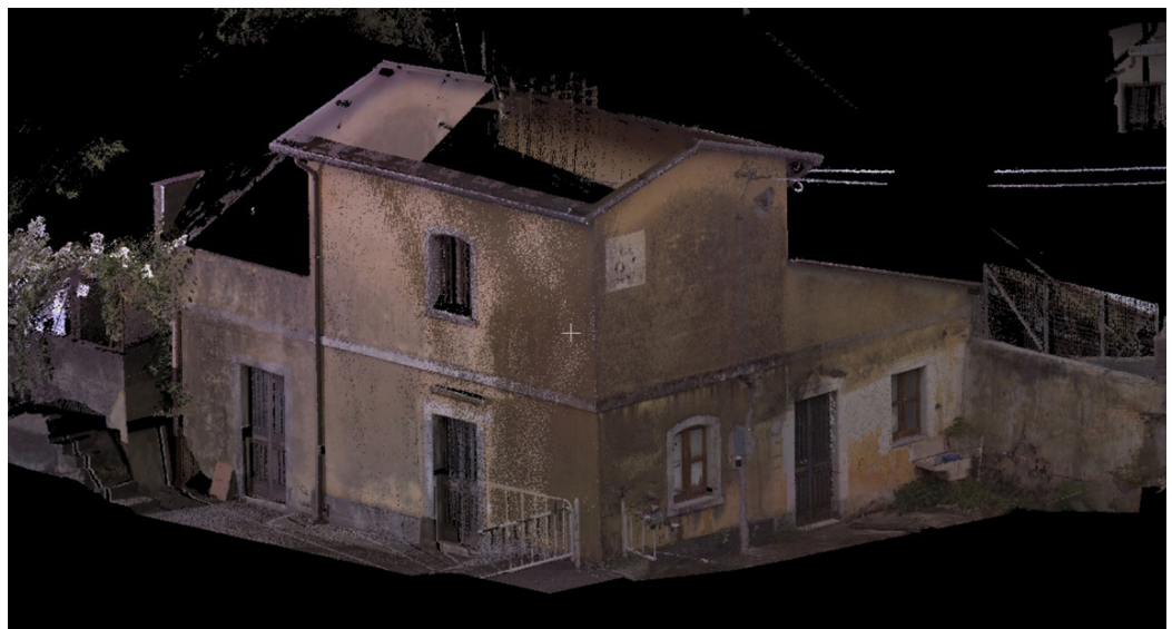
Fig. 12. The point cloud of the signalman's house 92 obtained through laser scanning survey.
