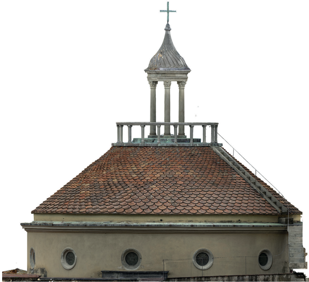
Fig. 8. Orthoimage of the exterior of the dome of the Sacristy, where you can see the unique structure with an Arabian-style dome positioned on the top (restoration by Sanpaolesi).
