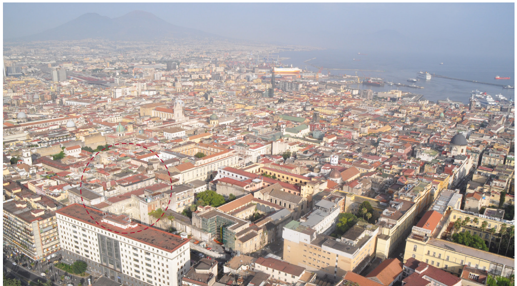
Fig. 1. Survey by the Benecon airborne platform, view of the City of Naples and focus on the Historic Pharmacy of S. Maria del Popolo degli Incurabili.
