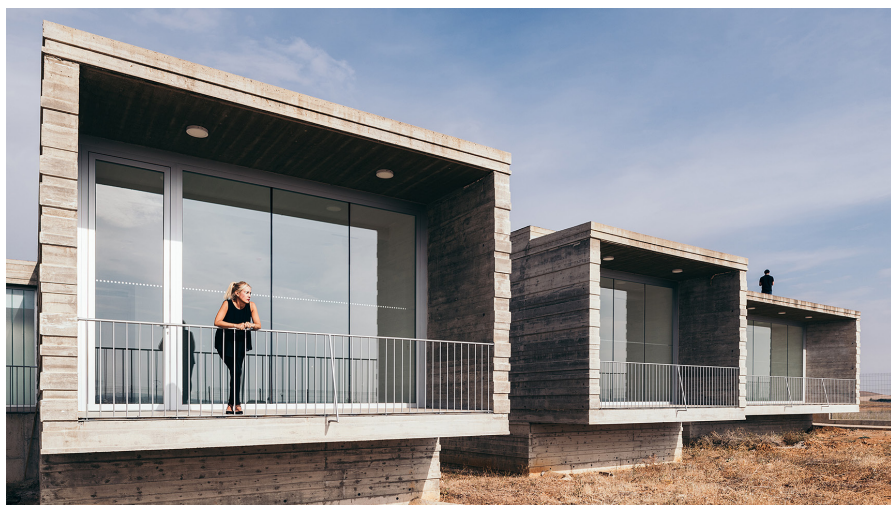
Fig. 1 – Alzheimer Daycare Center designed by studio VRA, Spain. Credits by Studio VRA.
