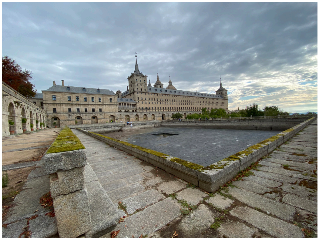
Fig. 11. The empty Friars' Pond showing the exceptional quality of the 16th century granite masonry covering walls and bottom (Photograph T. Abad 2021)
