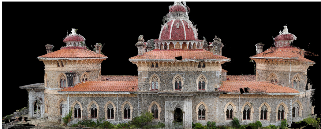
Monserrate Palace in Sintra. View of the north-east elevation of the dense point cloud obtained through the process of photogrammetry. (Graphic elaboration by Fabiana Guerriero)
