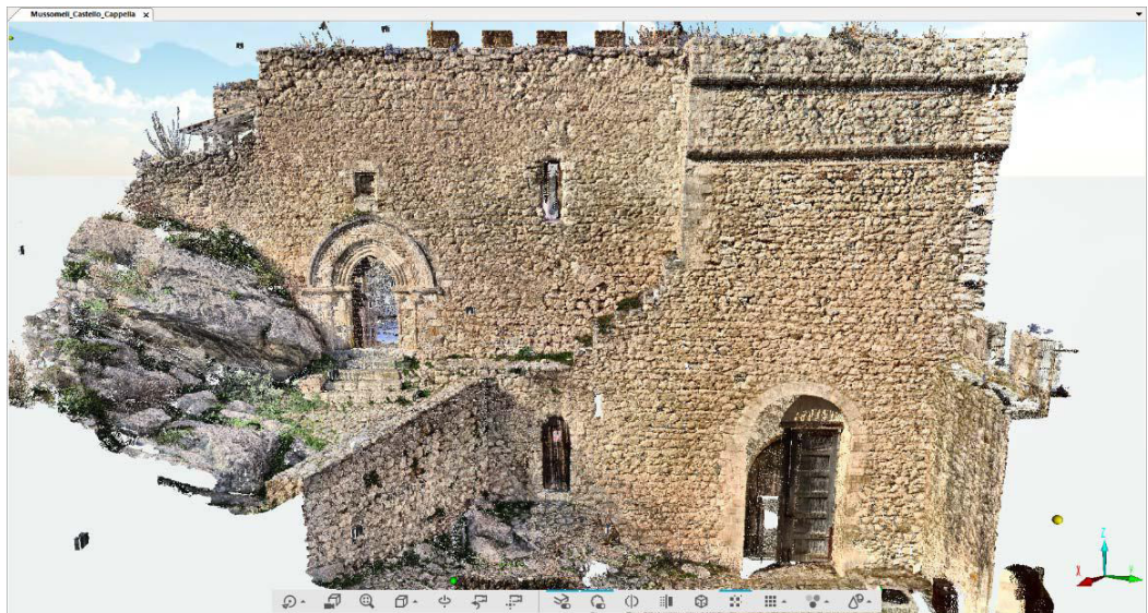
Fig. 05. Scan of the entrance side with the access portal and on the left that of the pointed arch chapel (Image by author).
