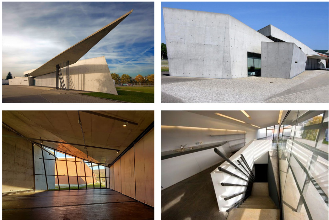
Fig. 2. Vitra Fire Station by Zaha Hadid (1990-1993).
