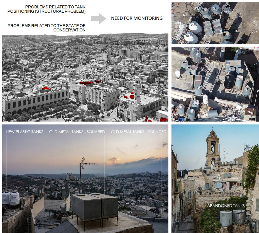
Fig. 1. Different tanks visible on the covering. The majority of surveyed tanks has a capacity of either 500 or 1000 litres, causing high load on the coverings.
