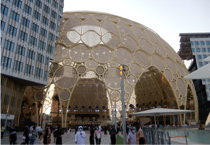
Fig. 1 - The Al Wasl Plaza, designed by Adrian Smith+Gordon Gill for Dubai Expo 2020, is an experimentation of multi-sensorial urban open space based on the coexistence of sounds, lights, shadows, wind flows. Photo by Filippo Angelucci, 2021.
