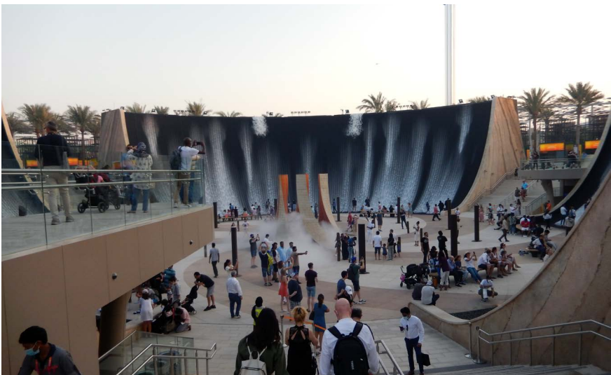
Fig. 2 - The Water Feature, designed by WET for the Dubai Expo 2020. Users are totally immersed in an experiential collective open space between water, vapour, and sounds. Photo by Filippo Angelucci, 2021.
